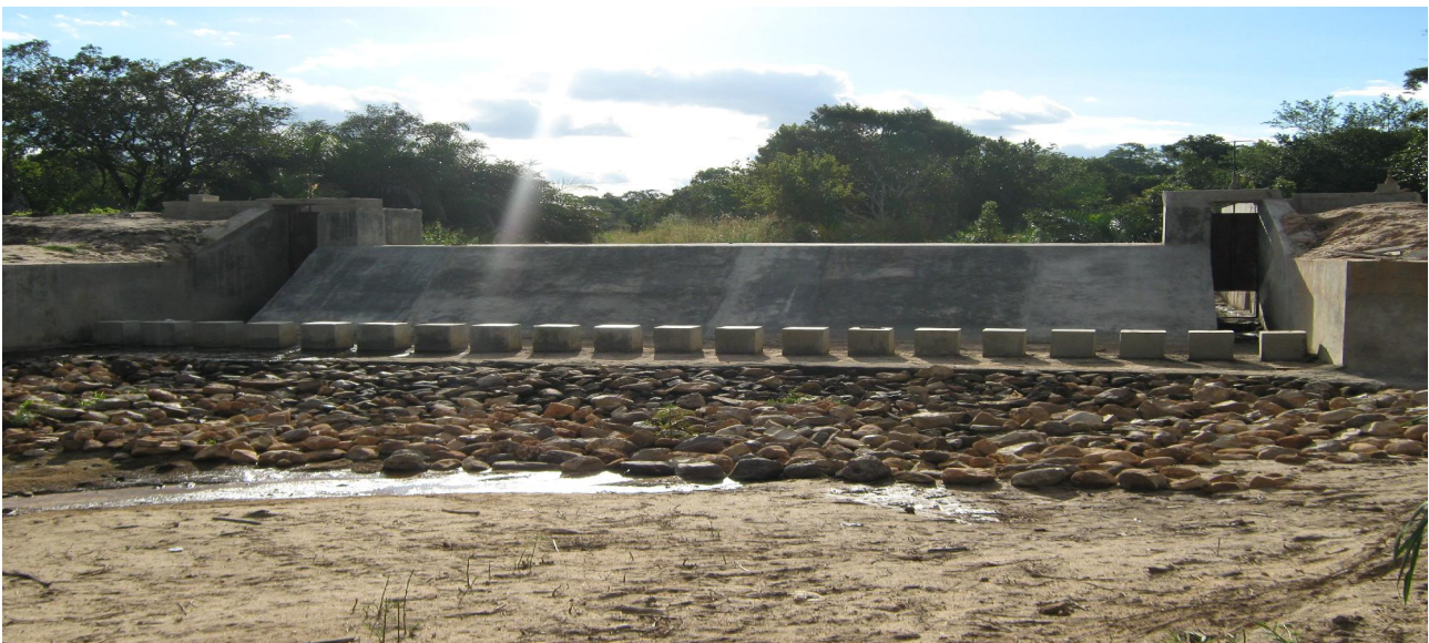
Fig13: Irrigation project in Ngongowele Village
