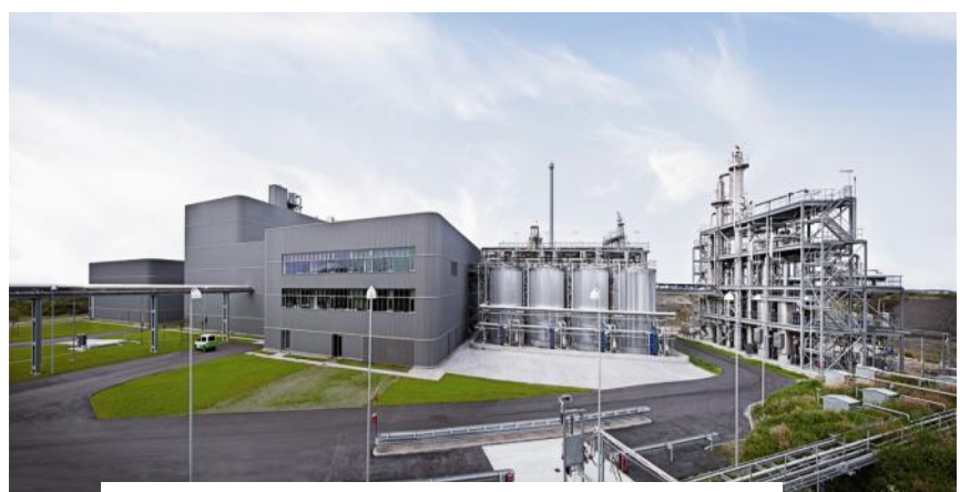
Inbicon biomass refinery demonstration plant
