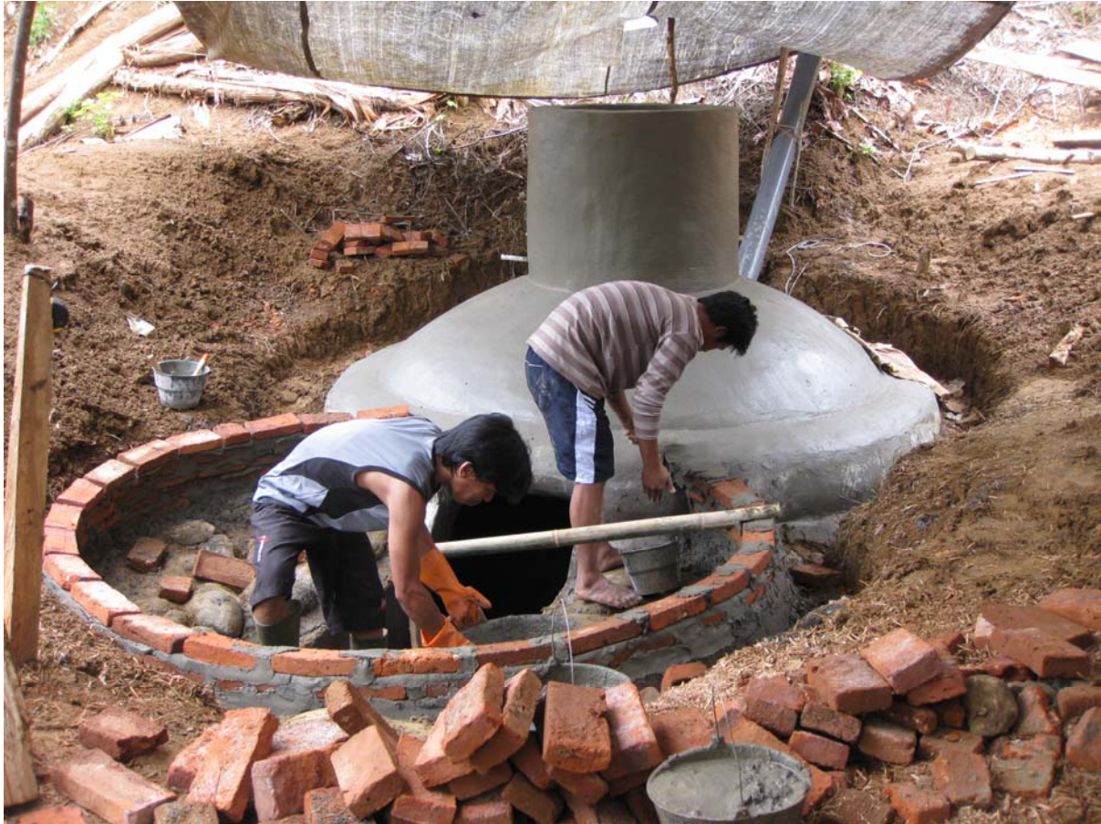
Payo Payo staff and Soga villagers building the Soga biogas digester in 2009
